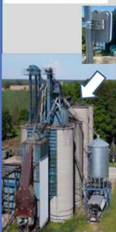
Installation of 60 GHz Network Installed In-Service Sept. 21, 2020
