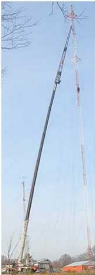
New 250' Tower Build - Completed Dec 2020
